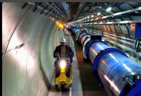
Blue tubes contain the two beam pipes and magnets at 1.8 degrees Kelvin
